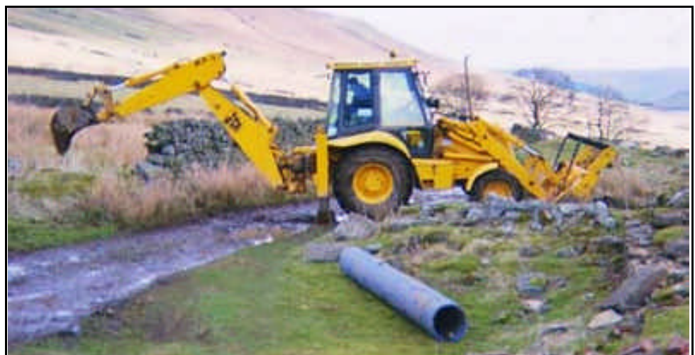
Photo: JCB repairing Deadmans Hill. (photo courtesy of Paul Sandlever.)
